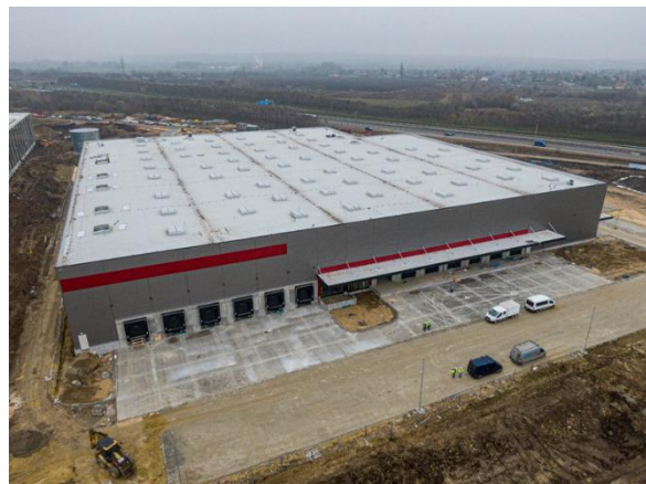
The new 12,000 m2 logistics center of Daniella Ltd. with a robotic warehouse system, which is the most developed and most innovative warehouse in the Hungarian electricity market / Source: Daniella Ltd./
